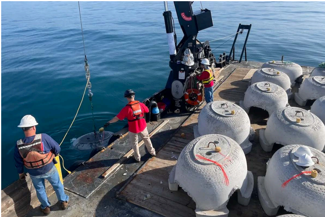
The first sea cave being lowered into the water. | Credit: Callie Fausey
